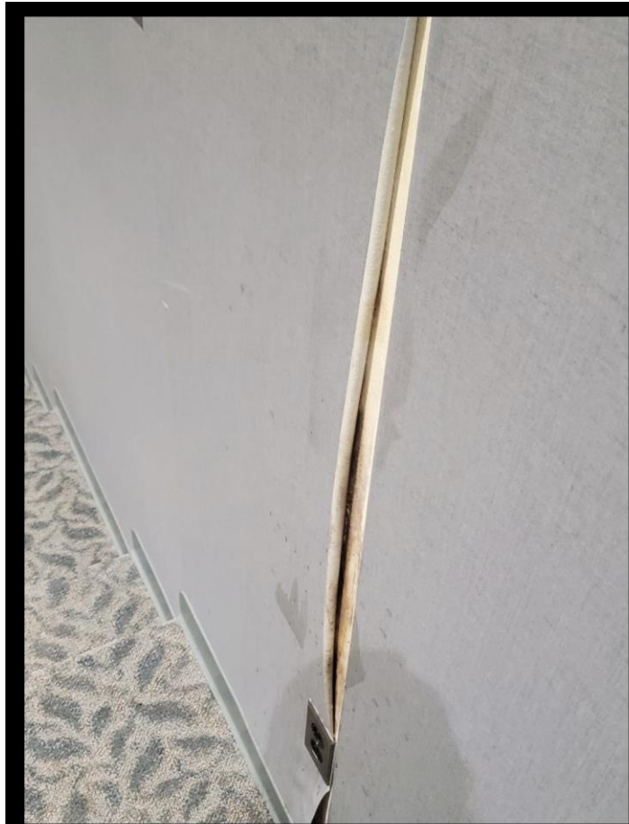
Peeling wallpaper around electrical socket, MEP building auditorium
